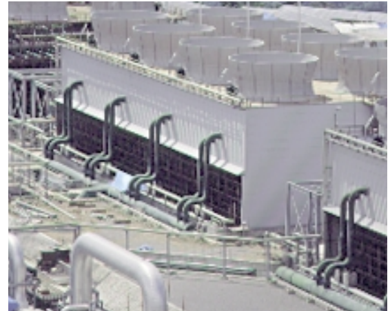
Fibercast's F-Chem large diameter filament wound piping, delivered to the Malitbog Geothermal Power Plant in the Philippines, the largest geothermal plant in the world. It is used in the plant's cooling water section.
